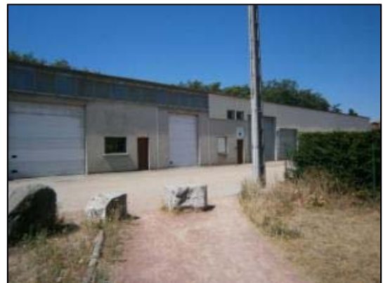
Centre technique municipal
