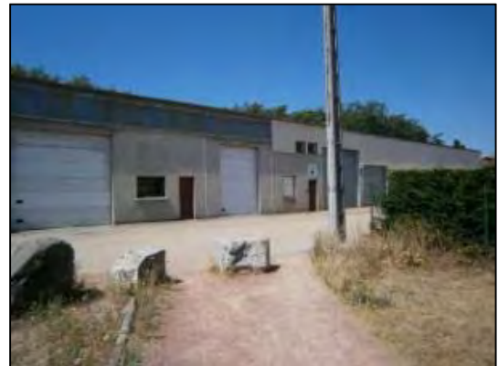
Centre technique municipal
